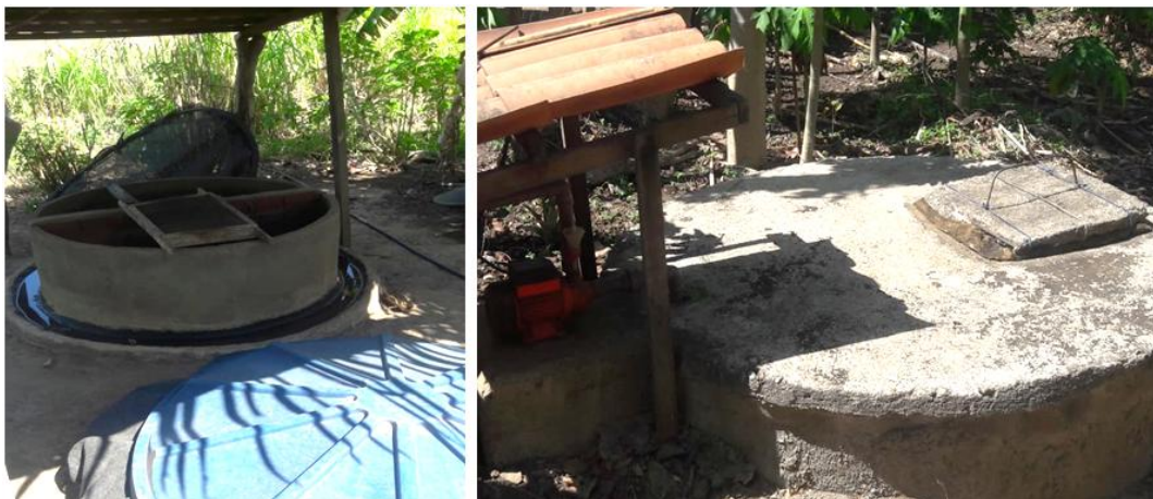
Figure 7 – Worm farm in Trapiá. Figure 8 – Well for the reallocation of gray water.
