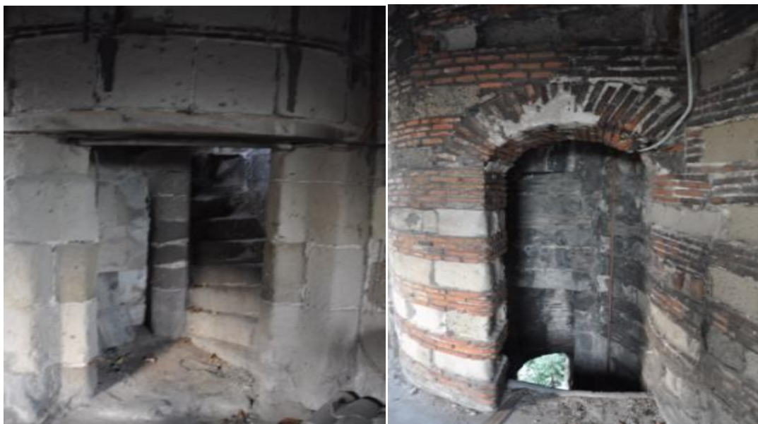
Fig.3. Manila. Santa Ana de Sapa. Tower. Spiral staircase
