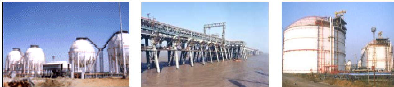
Figure 6: Jetties and Chemical Storage Tanks at Dahej
