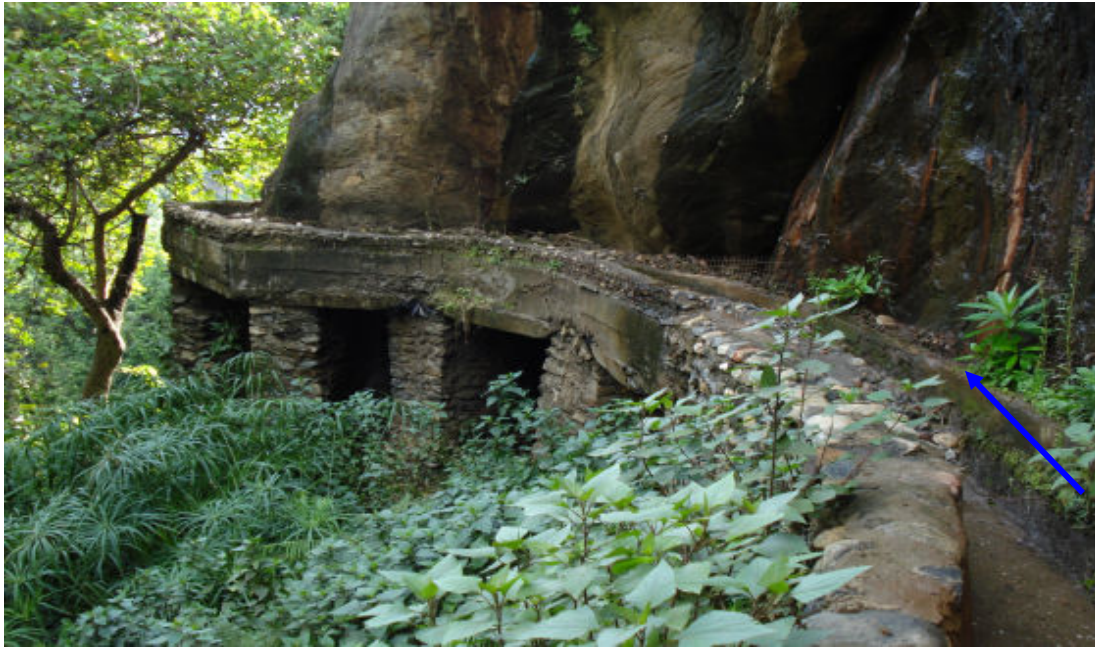
Plate 12. The Concreted Kapsyoi Furrow at the Baon Cliff constructed in 1980s
