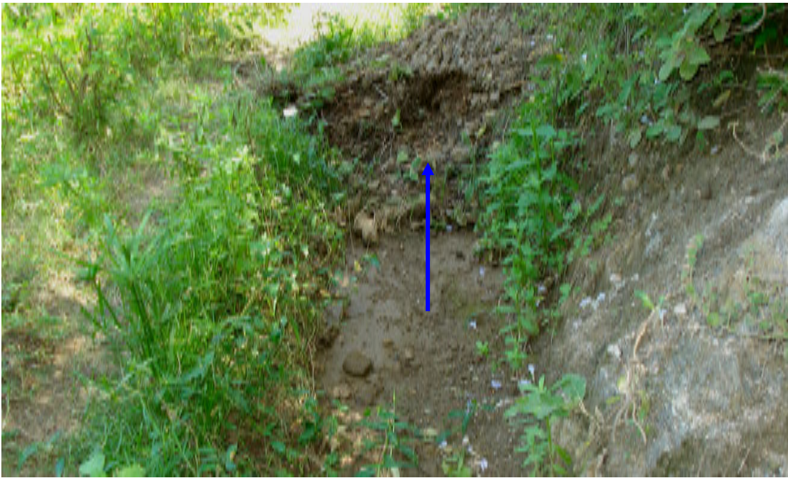
Plate 1 Blockage of the Kasukut Furrow by Mudslides
