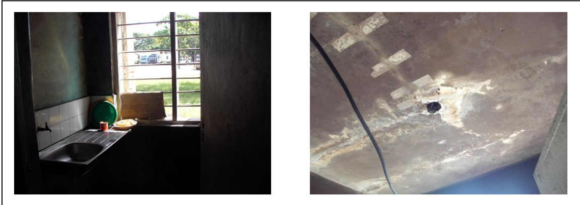
Figure 27. An abandoned kitchen as a result of a leaking sewage pipe through a ceiling in a flat at the Kilwa Road Housing Estate.
