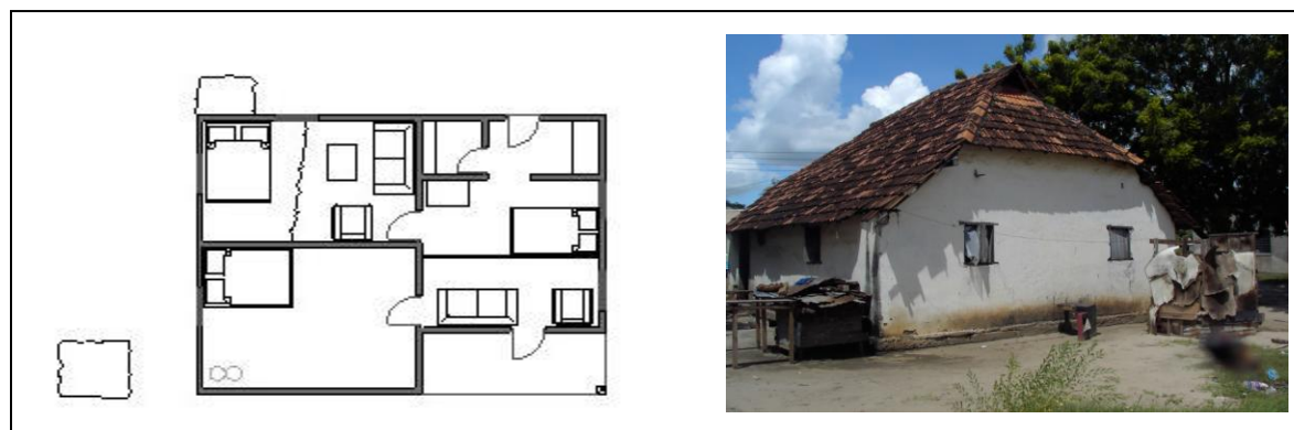
Figure 7. Mansard roofed house type with modified interior. A chipboard partition wall in the sitting room separates two families. These types of houses have deteriorated beyond repair. They have very small windows, which are inefficient for ventilation and enough light in the room.
