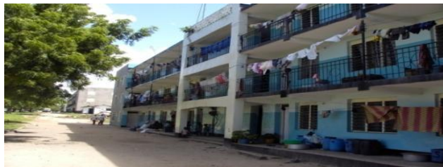
Figure 11. A reorganized staircase adjacent to a typical apartment in I-shaped block in Kilwa road housing estate
