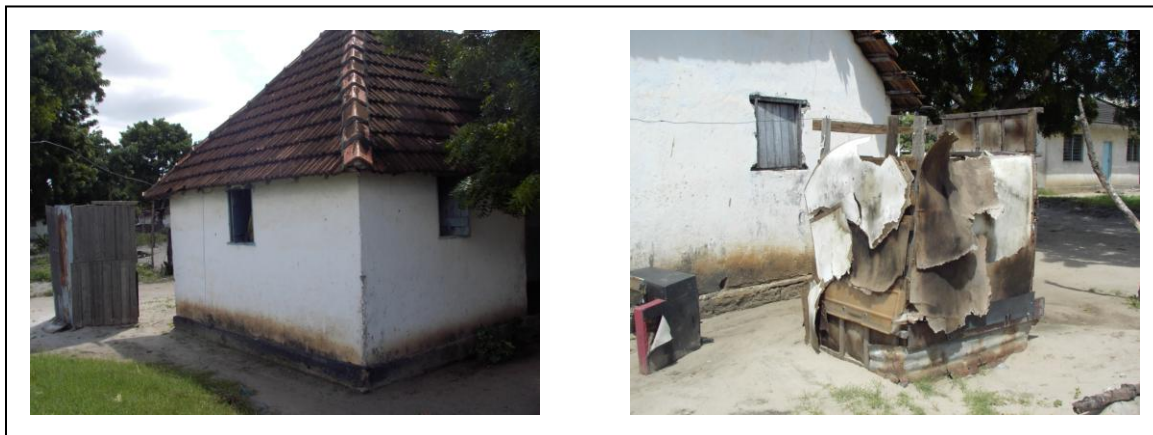
Figure 26. Pit latrines closer to the houses. Note the poor walling materials for the latrines.
