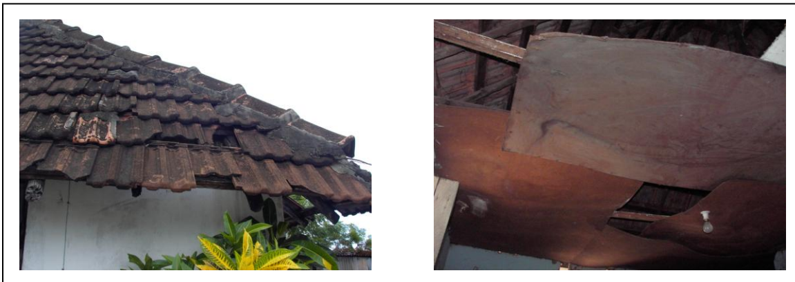
Figure 28. Dilapidated roof structure covering materials as well as ceiling board as observed in one of the visited houses at the Kilwa Road Housing Estate.
